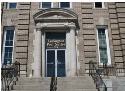
Pictured below: The building housing Dr. Lasnoski's office in Escanaba, MI
